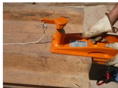
Drag the clip to the hole in the sheet pile.
