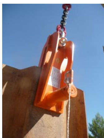
The sheet pile up and stable stall.
