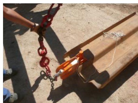
The sheet pile fixed, secure handling can be done.
