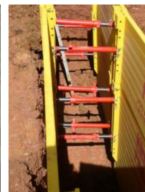
Care to preserve the contact between the plate and the ground
